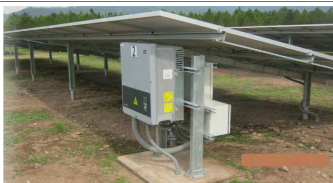
Figure 6.5: Typical Ground Mounted PV Array
