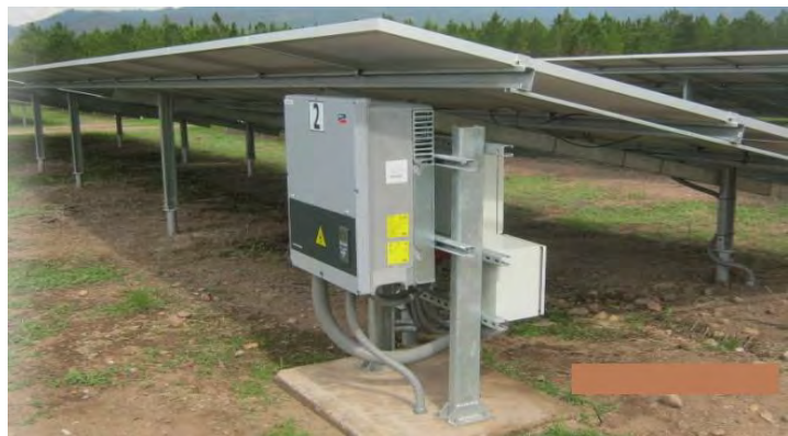
Figure 7.5: Typical Ground Mounted PV Array
