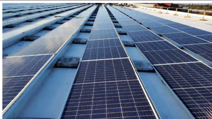
Figure 5.6: Typical Ballasted Roof Mounted PV Array
