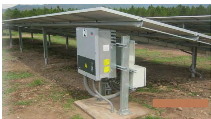
Figure 3.5: Typical Ground Mounted PV Array
