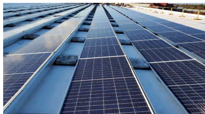
Figure 7.6: Typical Ballasted Roof Mounted PV Array
