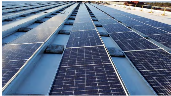
Figure 3.6: Typical Ballasted Roof Mounted PV Array
