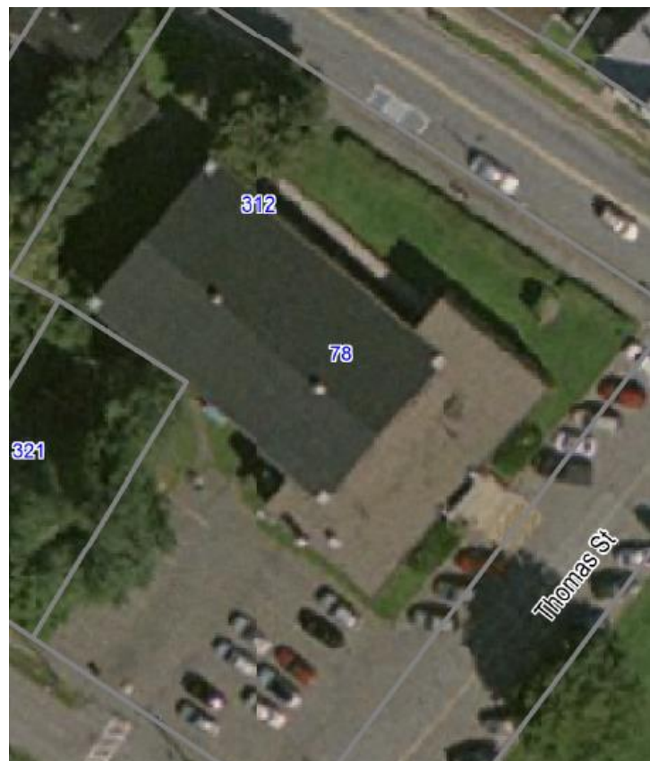
Figure 5: Orthophoto of Windsor Community Centre at 78 Thomas St.
