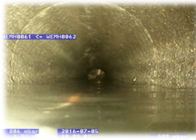
Pictures showing examples of pipe inspections.
