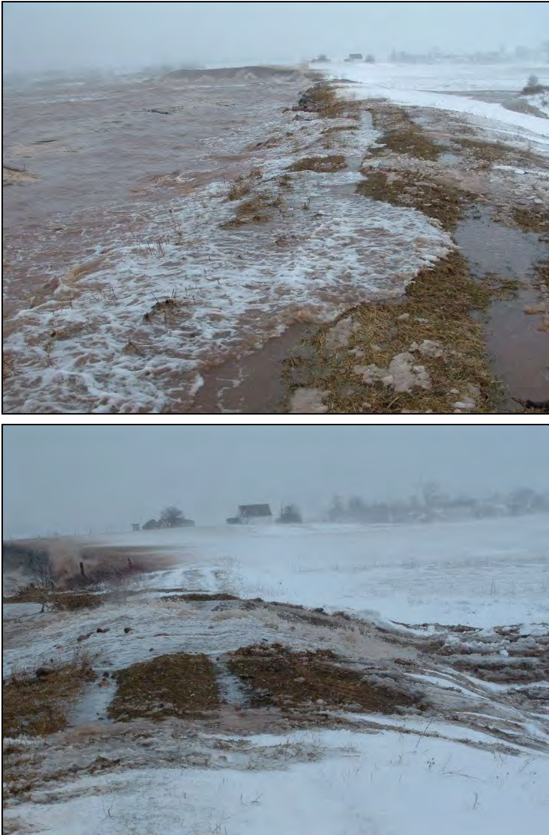
Figure 3: Storm impacts on Feb 1, 2006 at the Avonport Dyke. a) storm waves battering marsh; b) storm surge reached upper limits of dyke and dyke overtopped. Photo by T. Hamilton, 2006.
