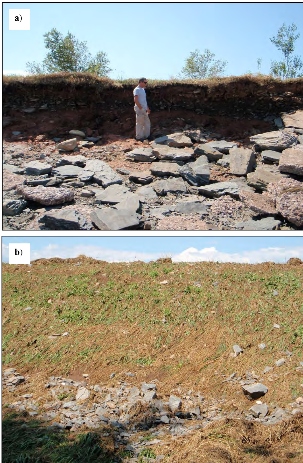
Figure 4: Impacts of Hurricane Bill on dyke at Noel in August 2009. a) erosion and undercutting of earthen dyke structure and removal of shoreline armouring, b) armouring rocks transported to the landward side of the dyke by wave action and overtopping. Photo by K. Carroll, 2009.
