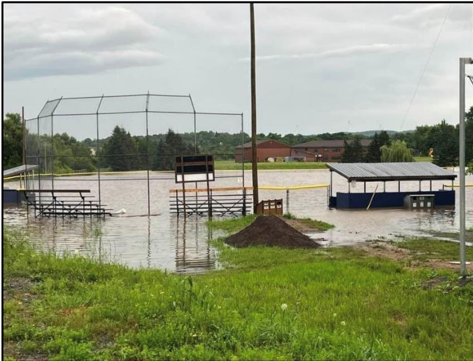
Figure 5: Aftermath of July 21/22, 2023 Rainfall Event – Flooding at the Coyote Park 'Big Field'
