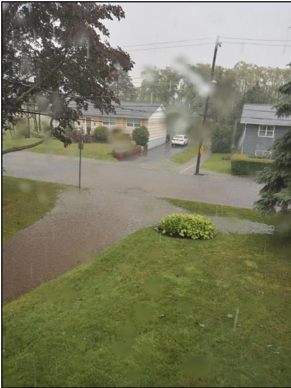
Figure 4: July 27, 2021 Rainfall Event, Swale by Civic #335 Flowing onto Tremain Crescent (Source: Local Tremain Crescent Resident)
