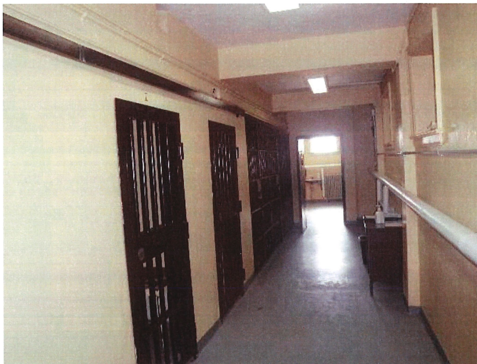
BASEMENT - CELL AREA
