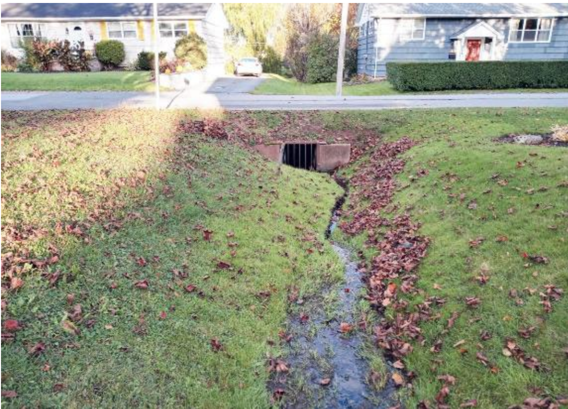
Figure 2 Ditch swale at 335 Tremain facing street and catch basin
