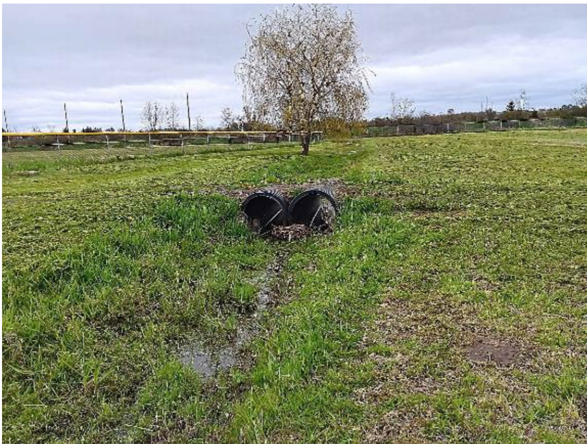
Figure 21 Marsh / Field Ditching and water back-up zone by the Ballfield and Elementary School Oct 2023
