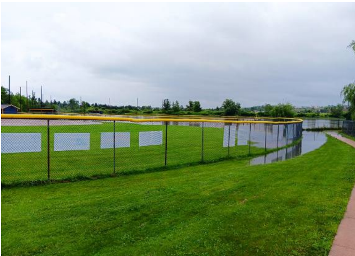
Figure 14 Ball field flooding across the street
