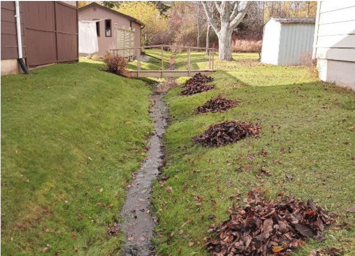
Figure 1 Ditch swale at 335 Tremain daily fall maintenance
