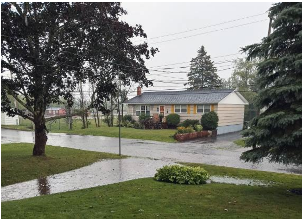
Figure 6 Culvert fully backed up causing floodwater to breach top of curb & flow across street
