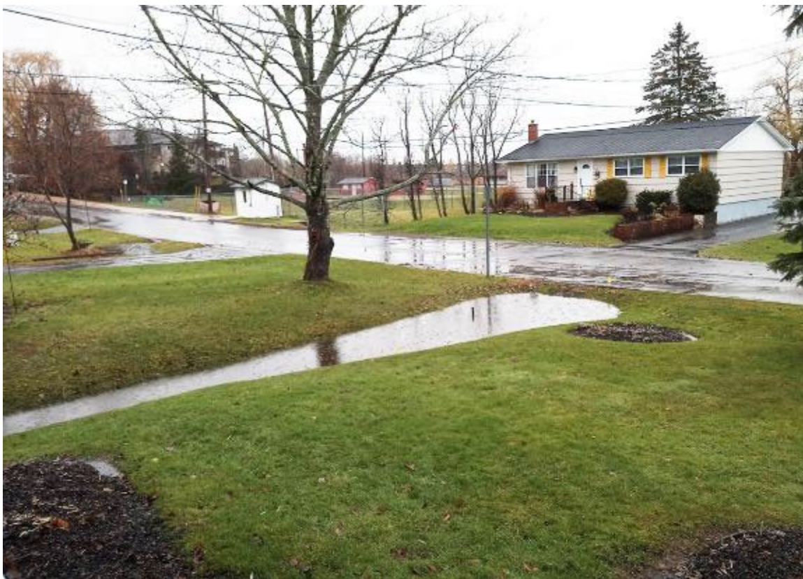
Figure 5 Flood water spreading across sides of ditch banks
