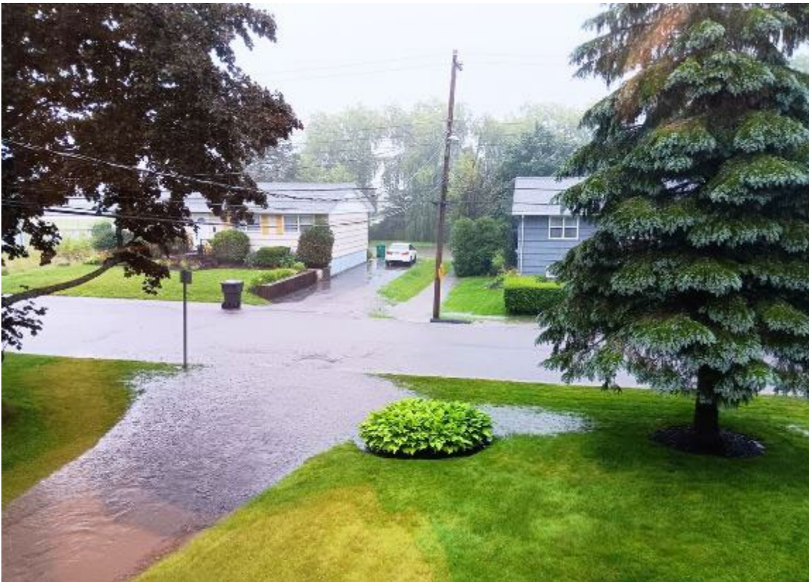
Figure 8 Culvert continues backing up and further flooding properties and street
