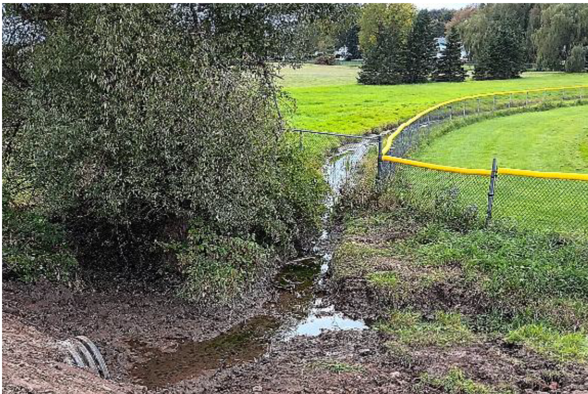
Figure 24 Culvert view from rail bed May 2024
