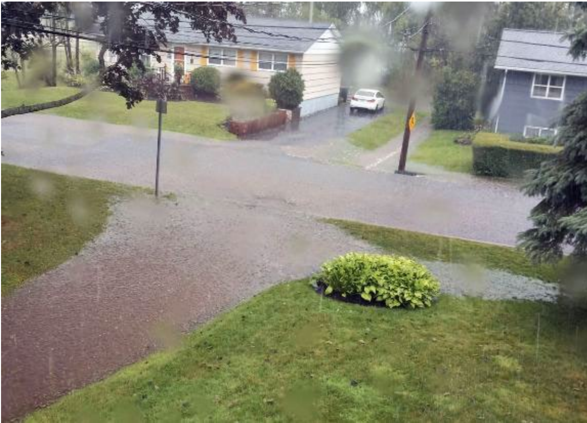
Figure 7 Culvert still backing-up floodwater across street and further onto sides of property
