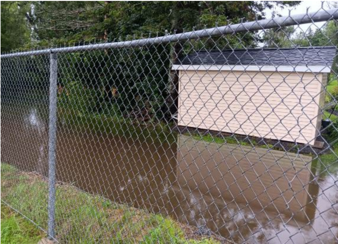
Figure 17 Flood water in drainage ditch (3 to 4 feet deep), from backed-up culvert and ditch on Tremain by ballfield and walking trail to elementary school.
