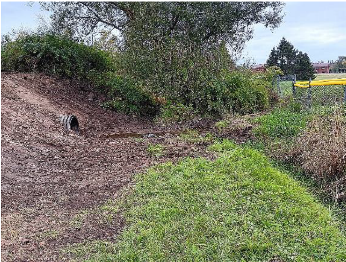
Figure 23 Culvert at the rail bed May 2024
