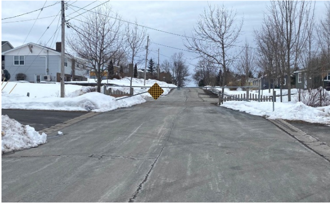
Photo 11-4: Underwood Drive Barrier
