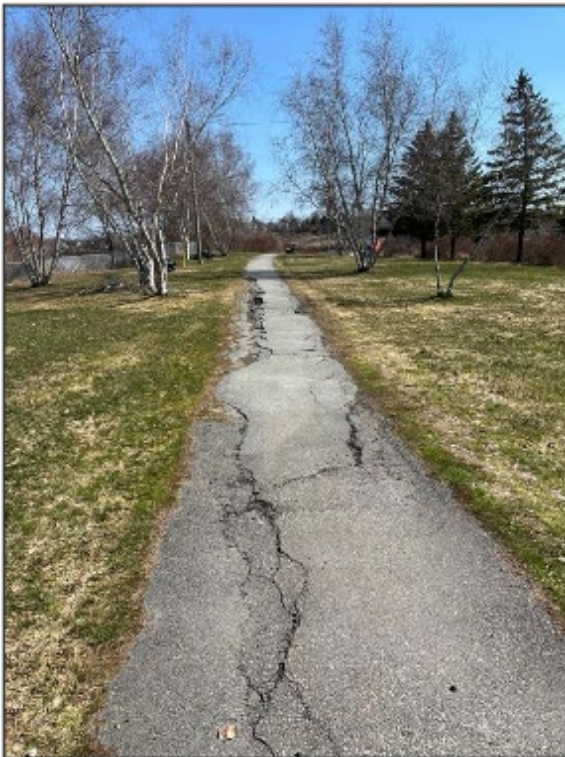
Figure 4. Example of Existing Condition
