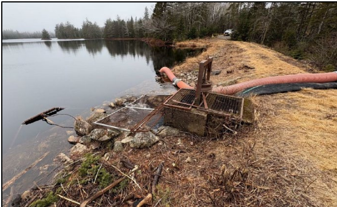
Figure 1-2. Existing Control Structure
