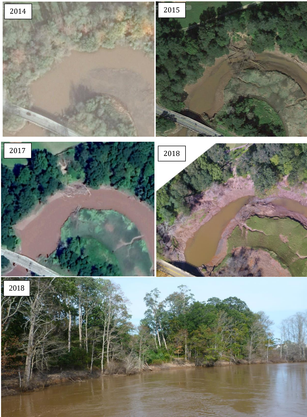
Figure 19 Progression of slope failure below Hantsport Community Center, 2014-2018 and landscape view at high spring tide, 24 September 2018.
