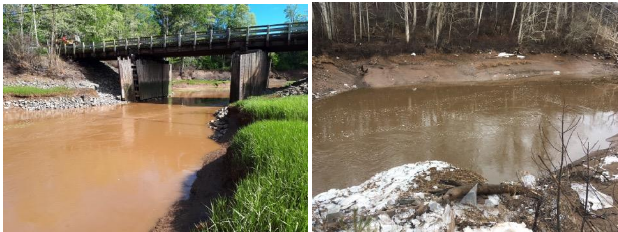
Figure 23 Highway 1 bridge at low tide from upstream marsh (left) and downstream eddies on outgoing tide (right). Photograph by CBWES Inc, 5 September and 7 February 2018.
