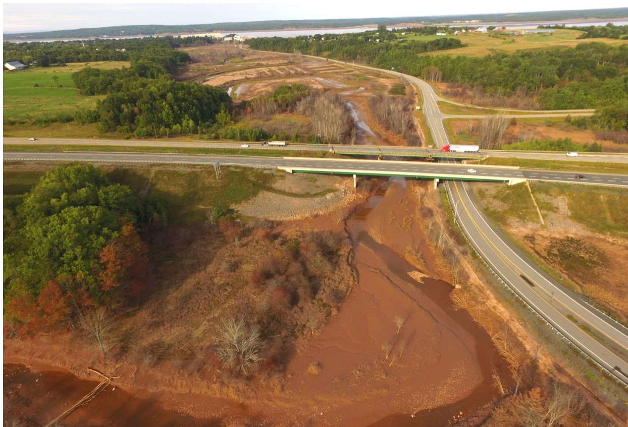
Figure 21 Highway 101, Exit 8 on/off-ramps. Upstream looking toward the mouth of the river. 5 September 2018.
