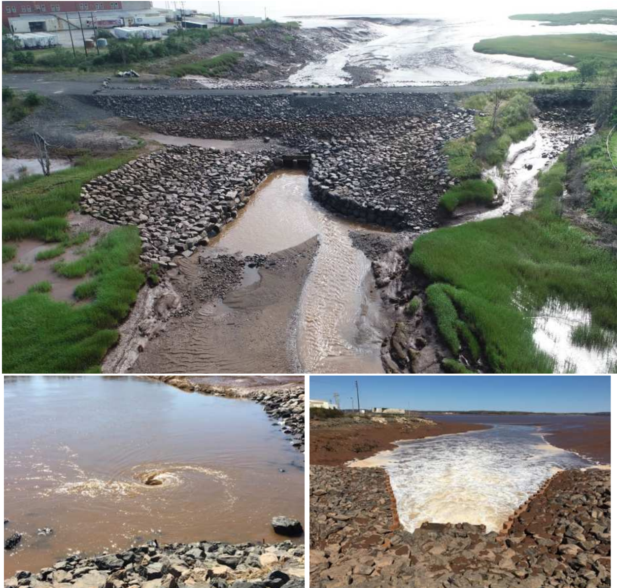
Figure 6: The causeway and double box culvert from upstream at low tide August 11, 2021 (Top); Discharge on falling tide downstream of structure with white water conditions for 50+ m (Bottom Right); Eddy upstream on falling tide (Bottom Left) both from May 20, 2020. All photos by CBWES Inc.
