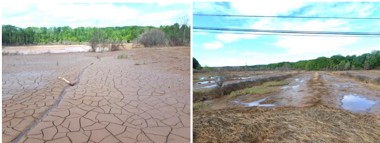
Figure 8 Heavy sedimentation in one of the main dales (left) and exposed crowns with dead grass visible (right). Photographs by CBWES Inc., 26 June 2018.
