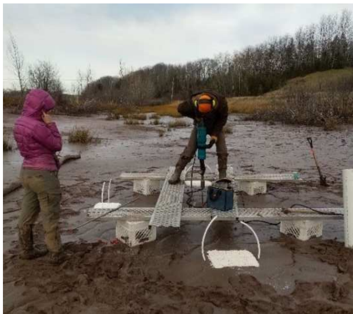
Figure 42: Installation of RSET 2 at HWR on November 27, 2019.
