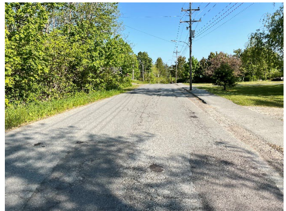
Asphalt & Asphalt Sidewalk Condition
