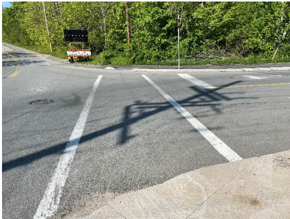
Bog Road Intersection (facing southwest)
