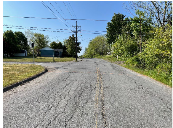
Rand Street (southbound view)
