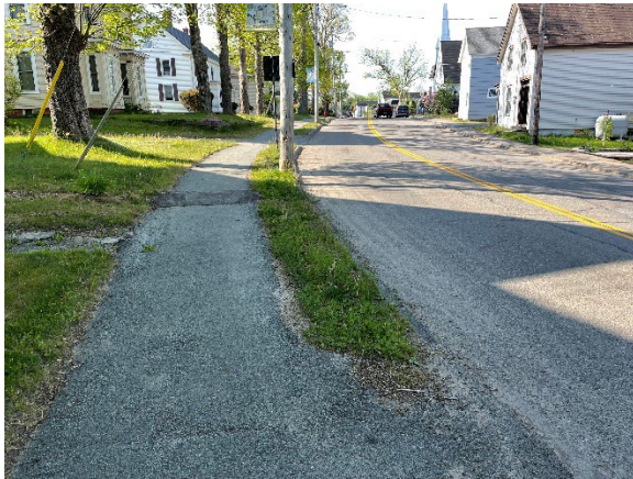
Asphalt & Asphalt Sidewalk Condition
