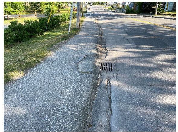
Asphalt & Asphalt Sidewalk Condition
