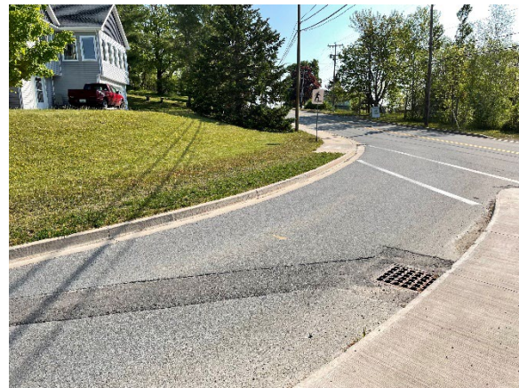
Holmes Hill Road Intersection (facing east)
