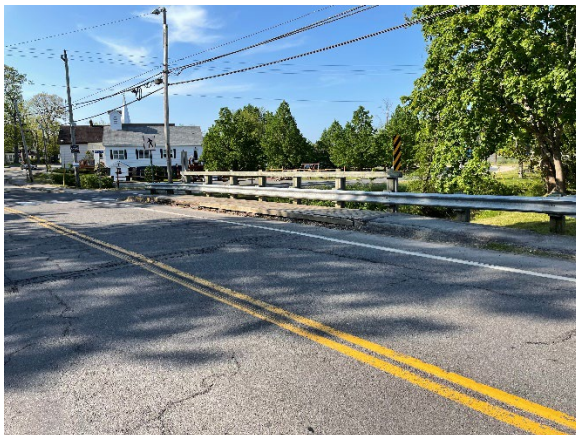
Willow Street Bridge (NSDPW jurisdiction)
