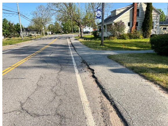
Asphalt & Asphalt Sidewalk Condition
