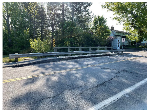
Willow Street Bridge (NSDPW jurisdiction)
