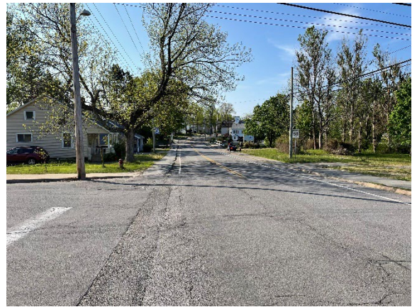
Main Street North (southbound view)
