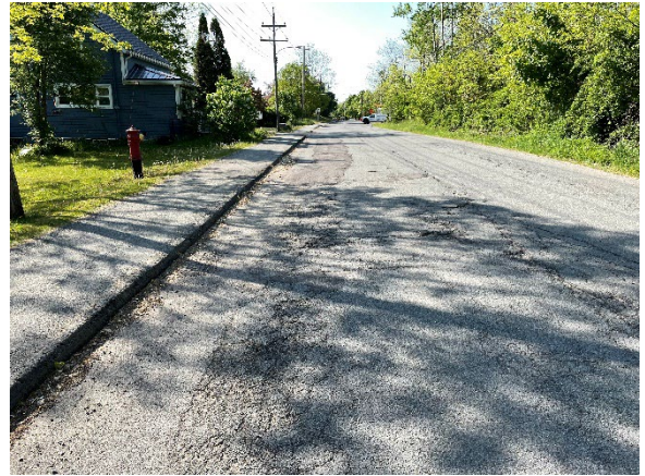
Asphalt & Asphalt Sidewalk Condition
