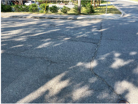
Asphalt & Asphalt Sidewalk Condition
