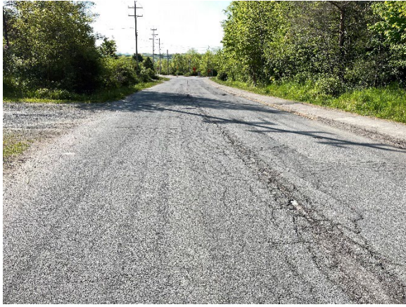
Asphalt & Asphalt Sidewalk Condition
