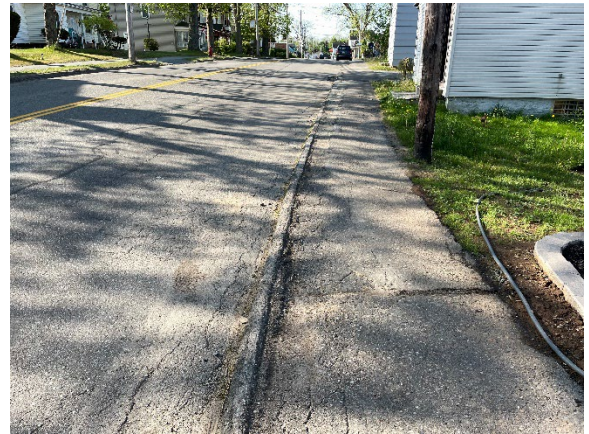
Asphalt & Asphalt Sidewalk Condition
