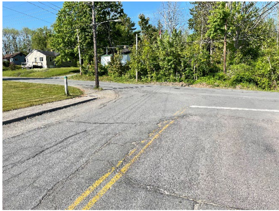
Asphalt & Asphalt Sidewalk Condition
