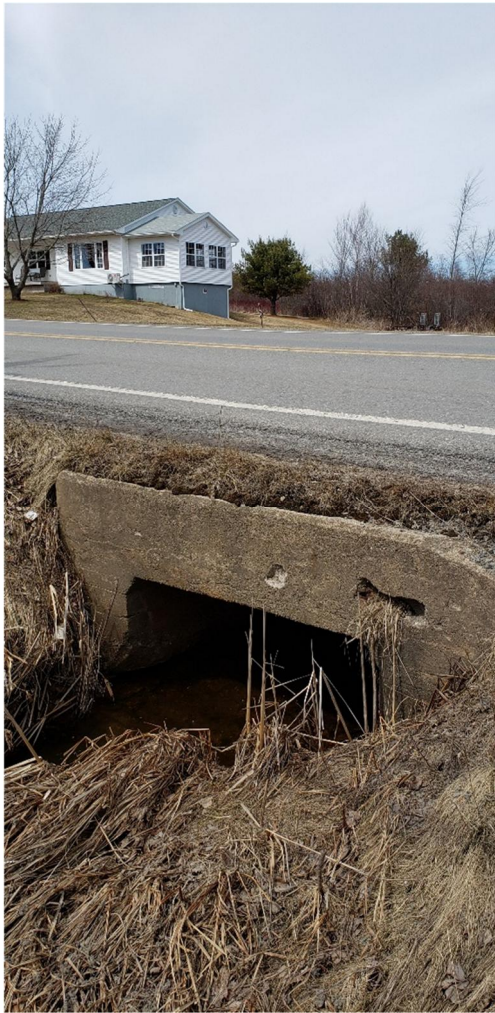
Figure 3-6: Downstream Side of Box Culvert Crossing at Civic #4627 on Highway 1
