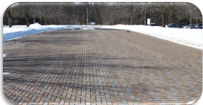
Figure 7-6: Installed Permeable Pavers in Winter (trca, 2015)
