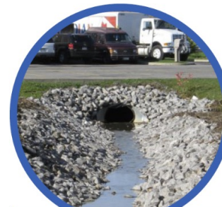
In-Street (Cross) Culverts
