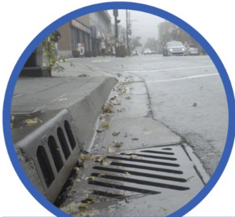
Storm Drains (Catchbasins)
