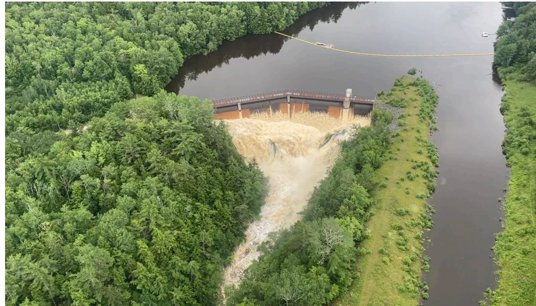
NS Power Dam – Falls Lake
