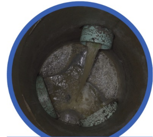
Buried Pipes & Manholes
