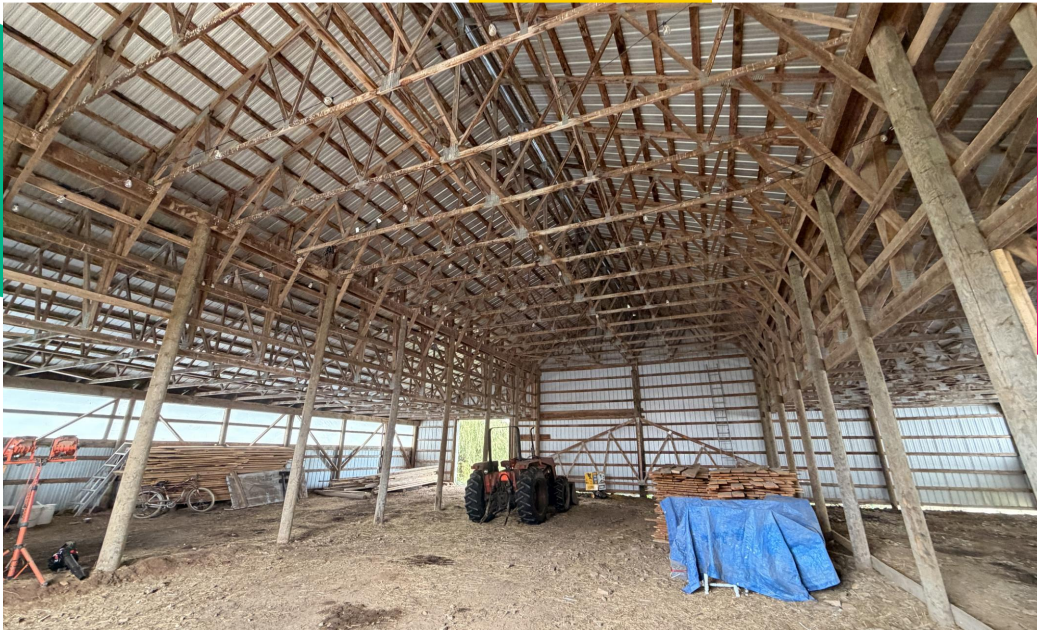
Existing barn, interior
