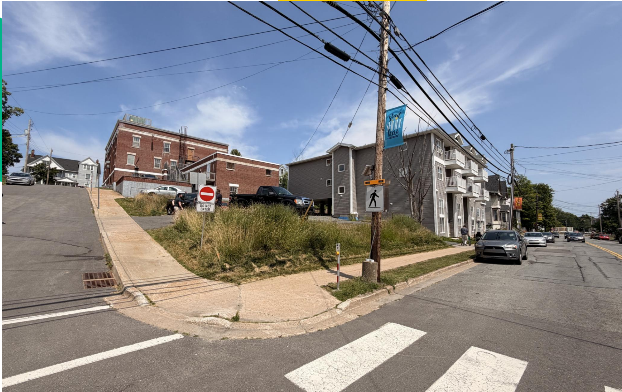
View of the existing buildings from Gerrish Street
