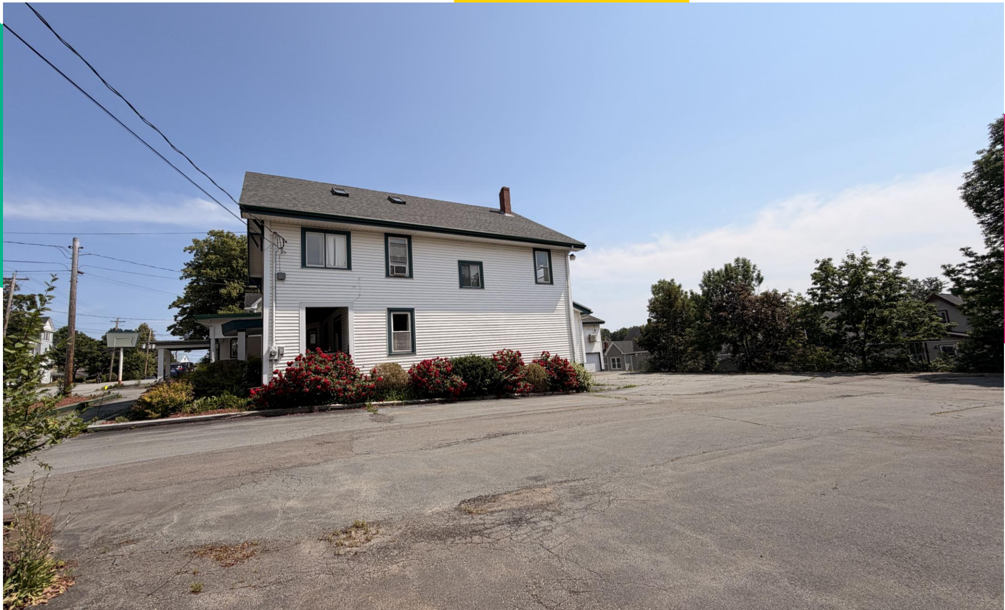
View of the existing buildings from the parking lot.
