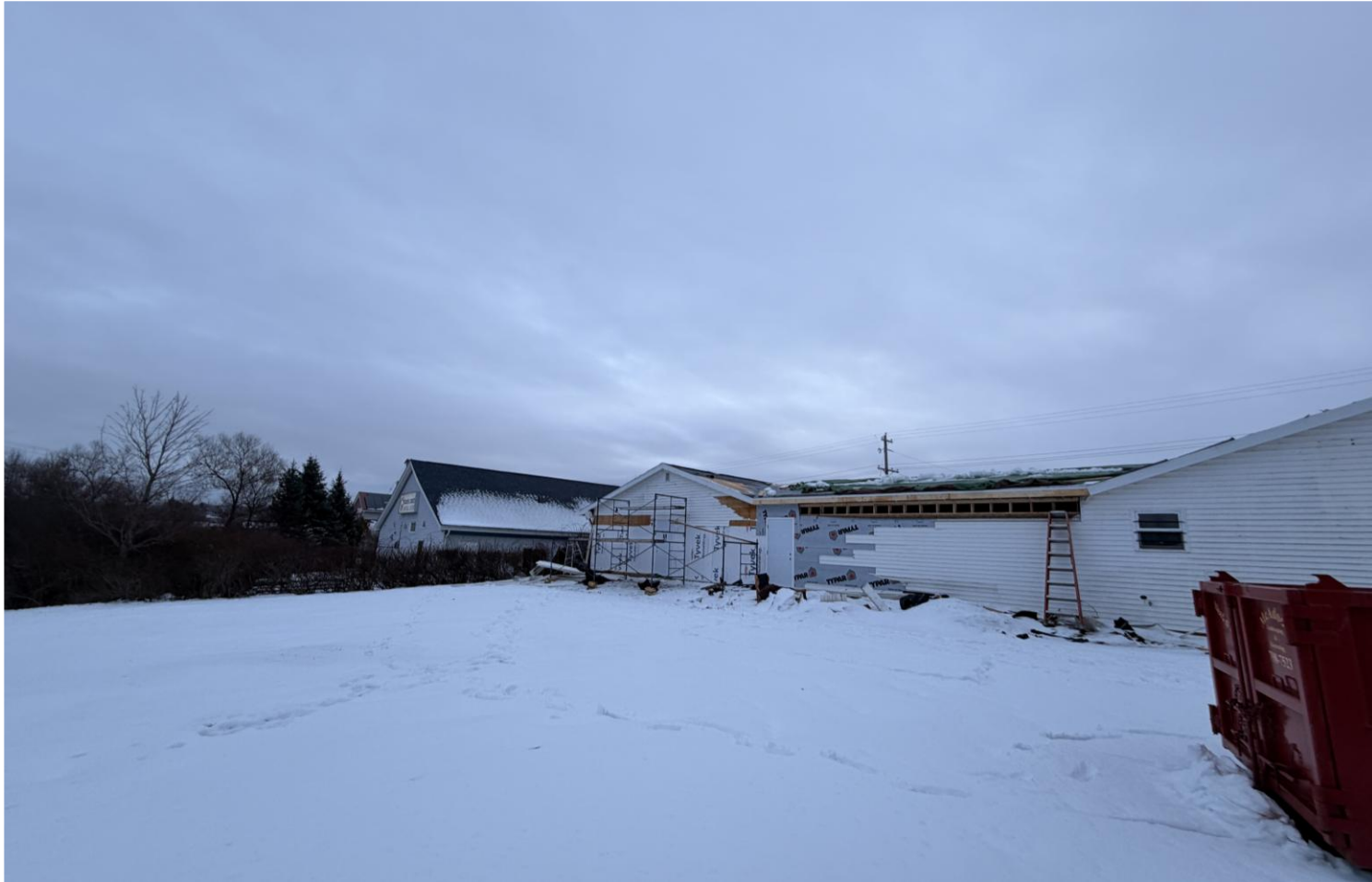
View of the rear yard of the subject lot
