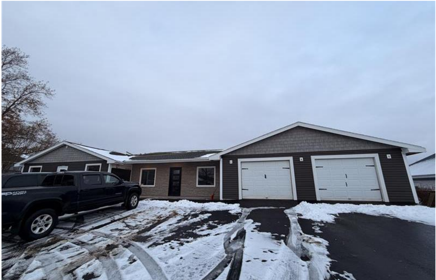
View of Subject Lot fronting Highway 1
