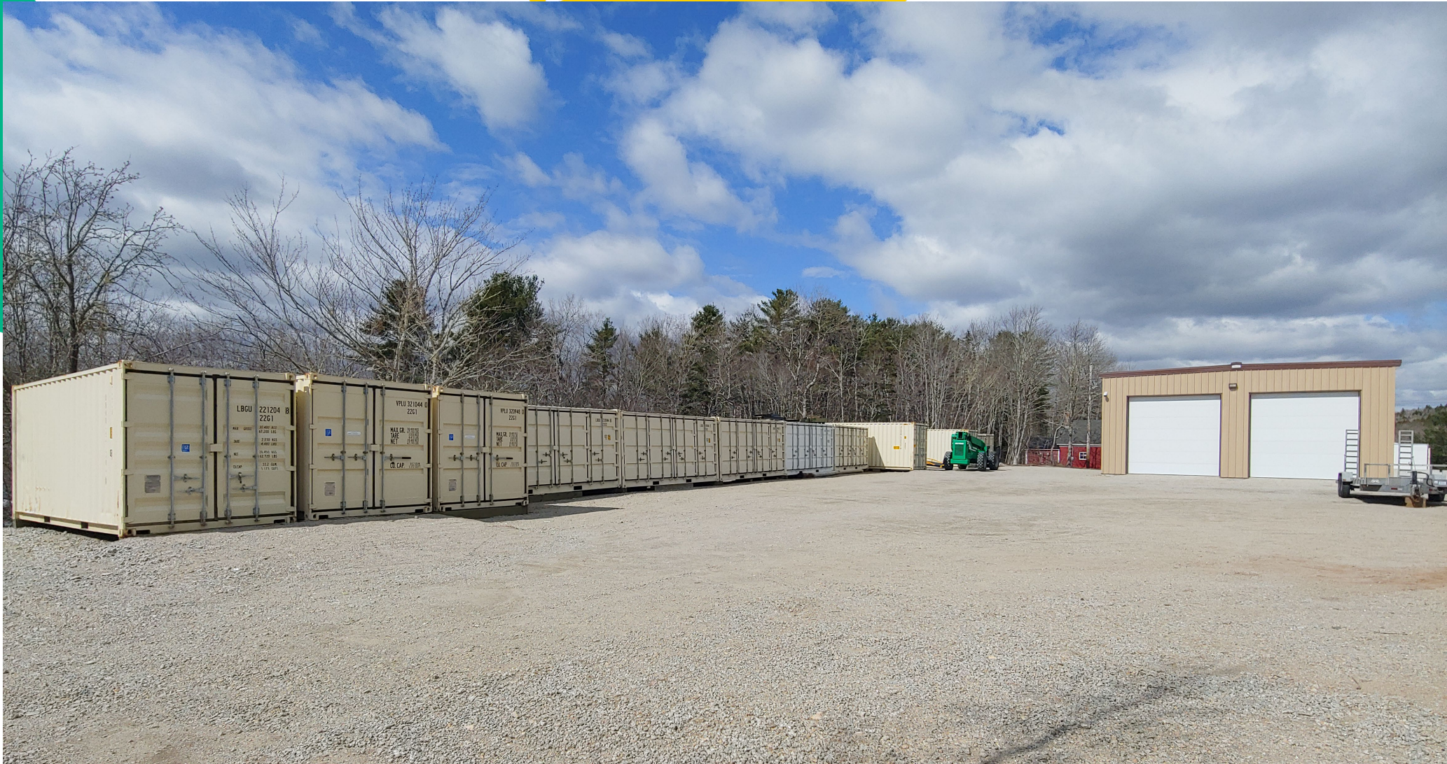
View of Subject Lot from front access point
