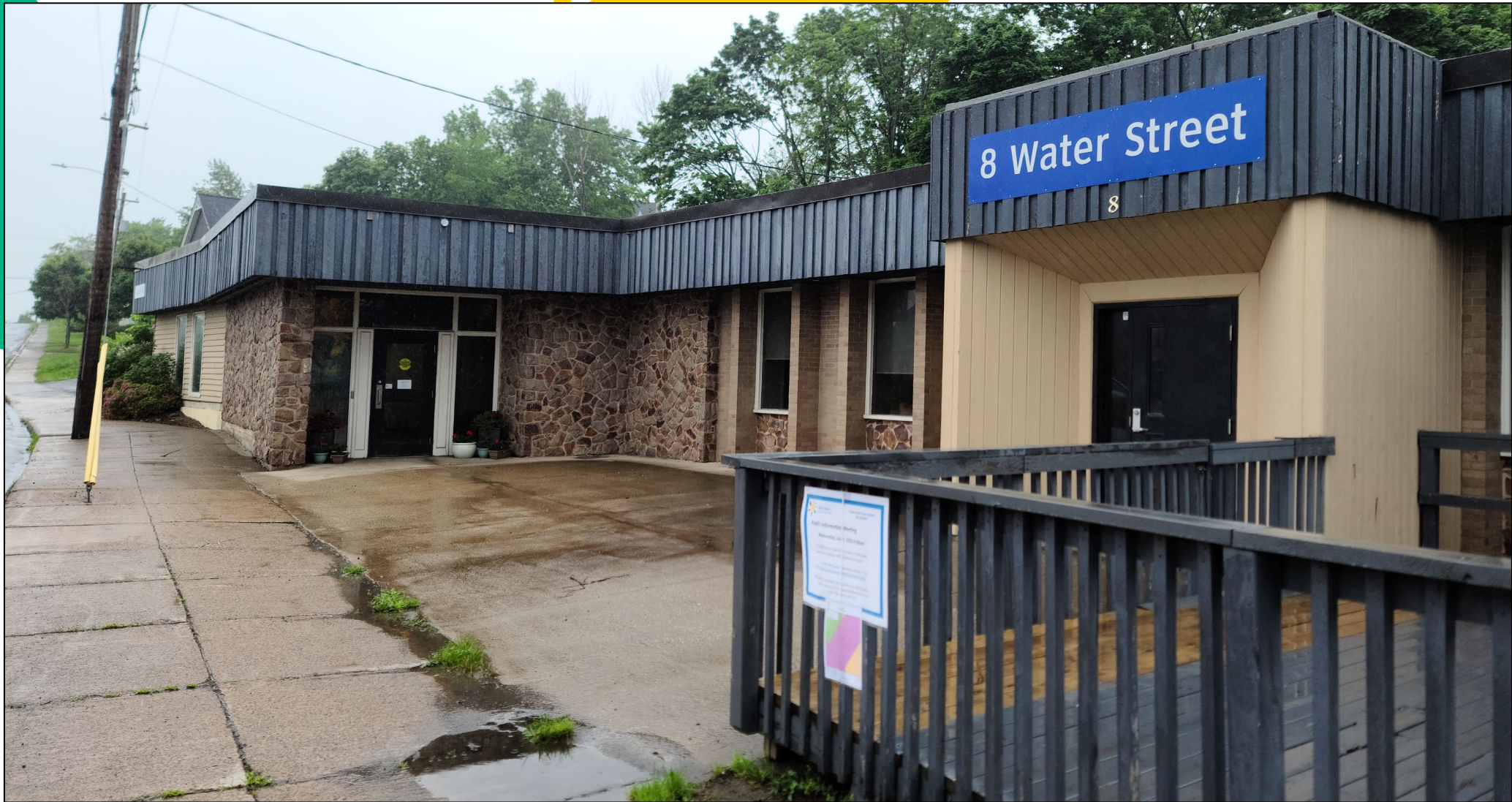
View of Subject Lot from Upper Water Street
