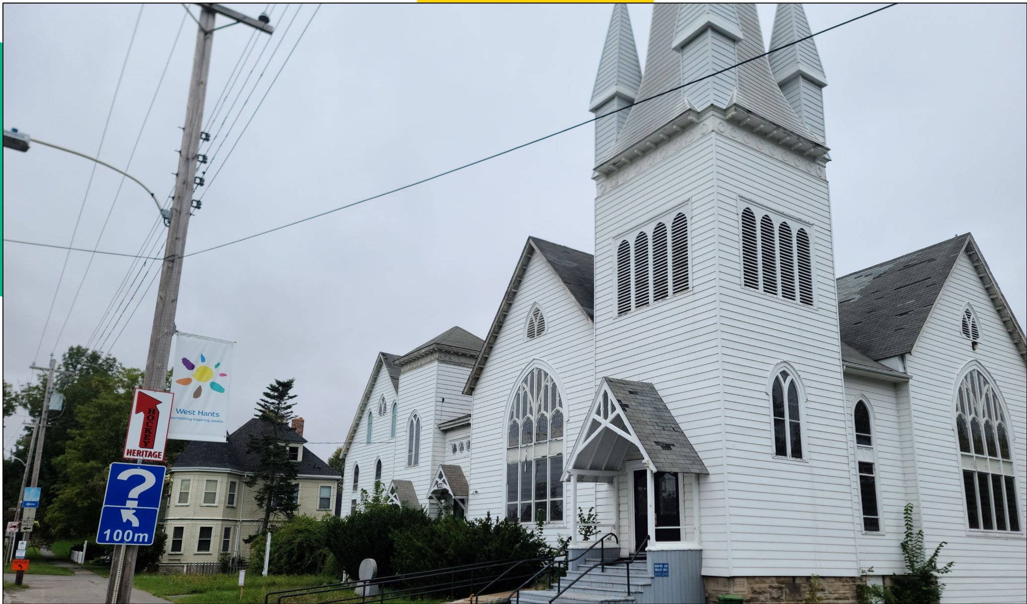
View of Subject Lot from King Street
