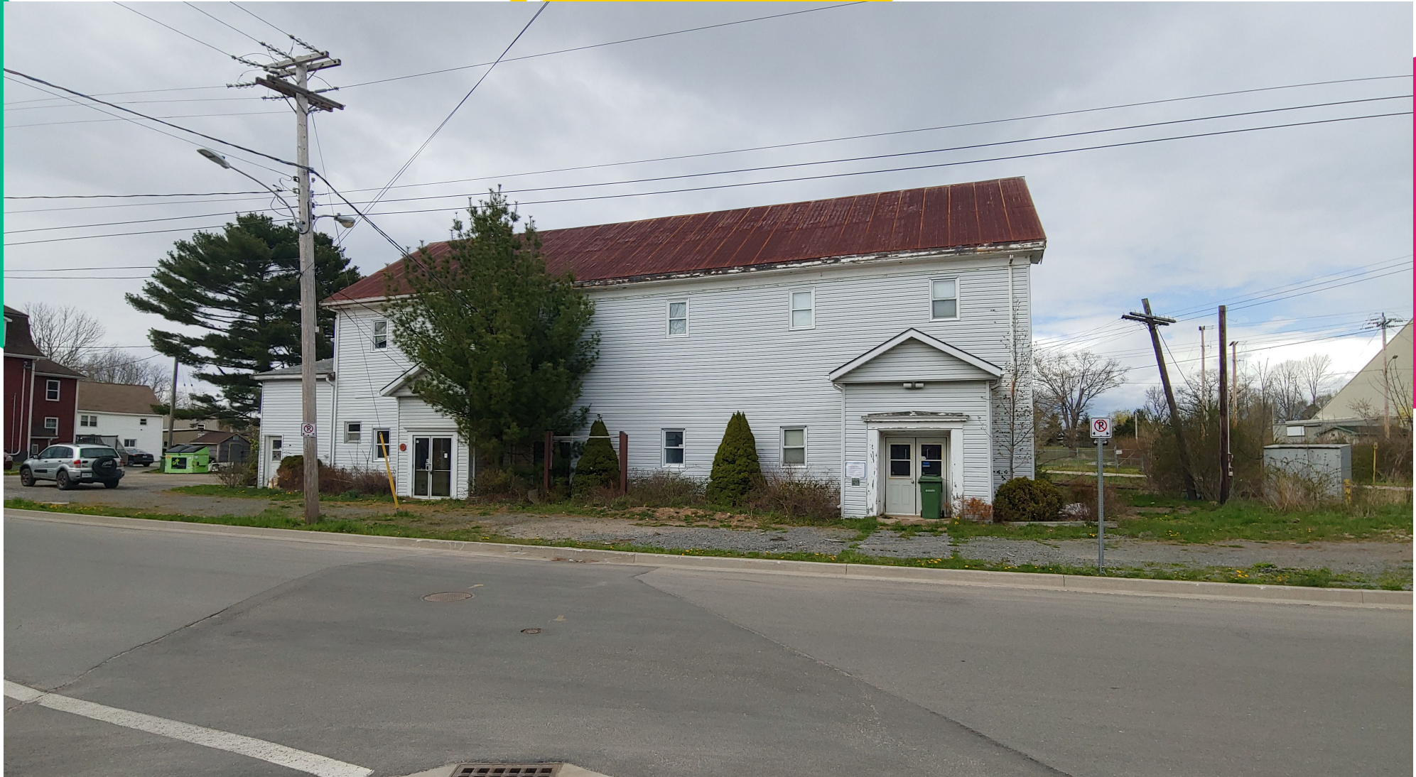
View of Subject Lot from William Street
