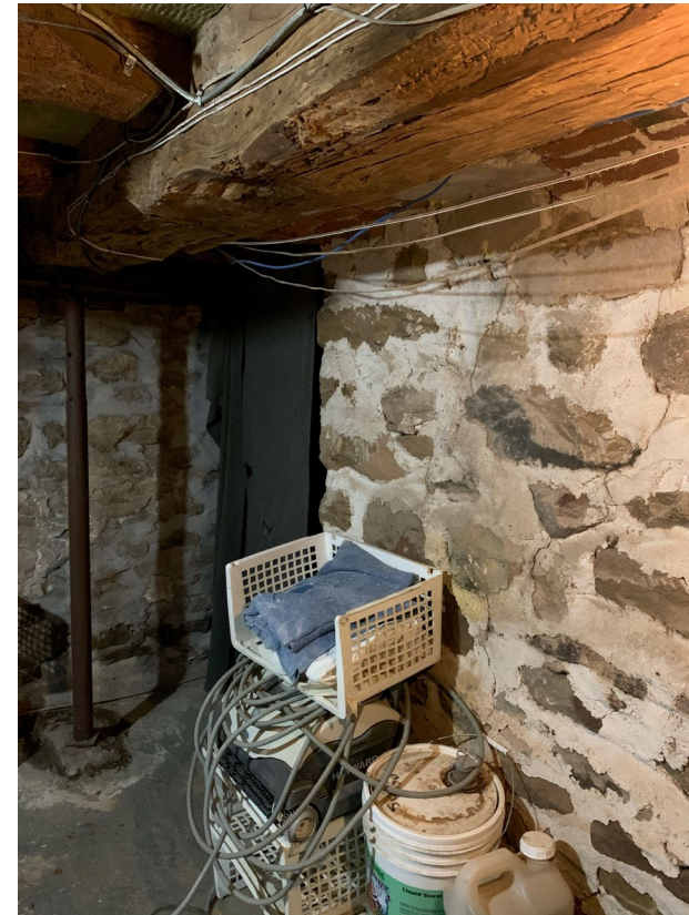
Original stone and mortar foundation
