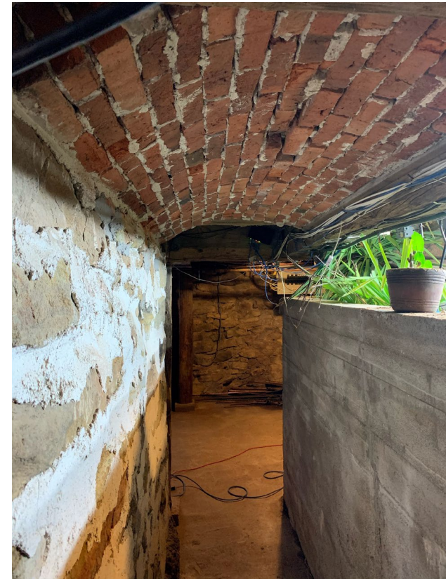
Original stone and mortar foundation
